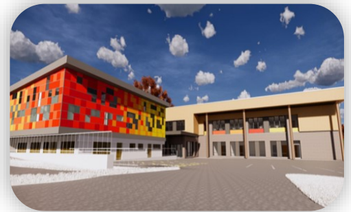
Health and Wellbeing Hub under development in Llanedeyrn
